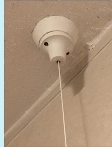
You might find a **pull switch** in the bathroom to turn the light on.
